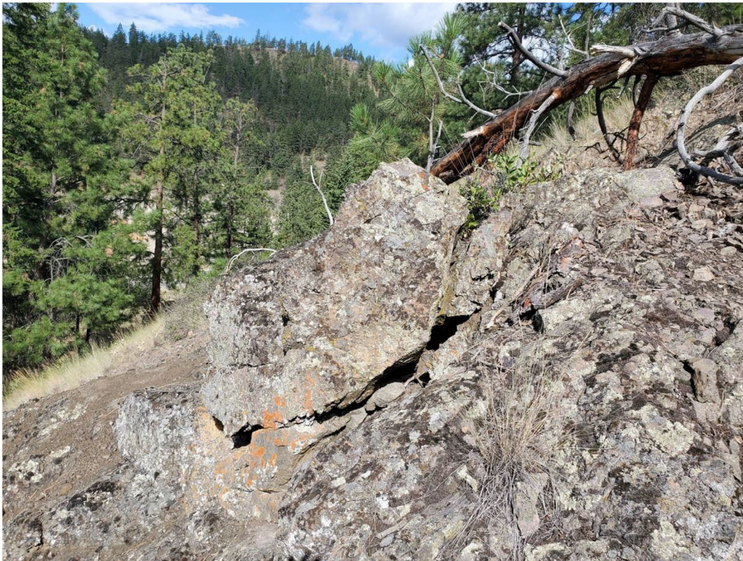
Figure 5B. Loose rock near the centre of 1490 Cara Glen Way.
